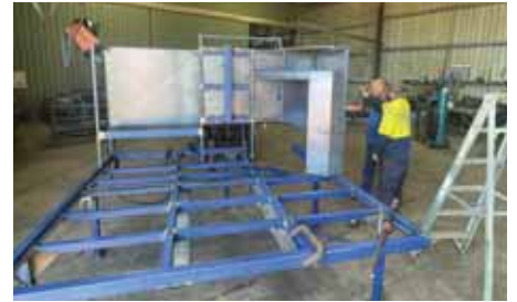
A sheep delivery module under construction at RW Engineering.
