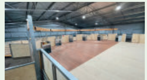
A new shed at 'Doreenup' at Kojanup built for the Eyres family by Chippy Chad & Co Construction, based on the AWI Shearing Shed Design.
